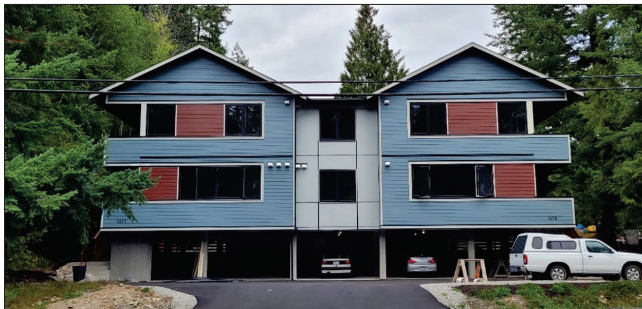
1477-1479 Depot Road, Squamish – 14 micro-suites
